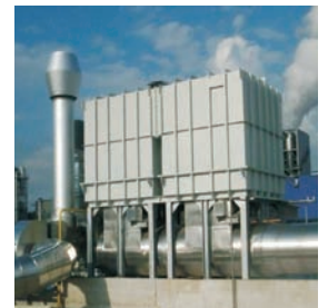
Regenerative thermal oxidiser
